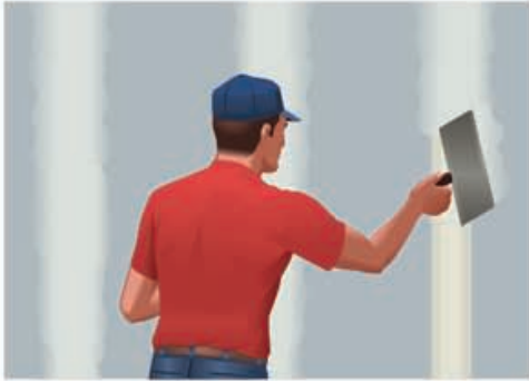
N1709P69007C*-O (Applying Joint Compound)
